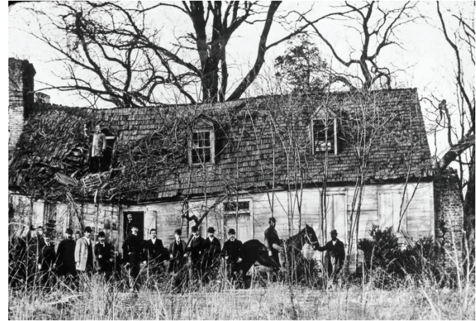
Members of the AOI assemble in front of the David Burnes cottage which stood near 17th & B Street, NW (c. 1885) [HSW Collection]
