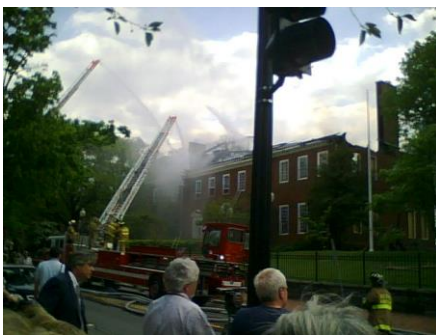
DC Fire Department Pours Water on the April 20, 2007 Fire That Consumed the Georgetown Branch Library
