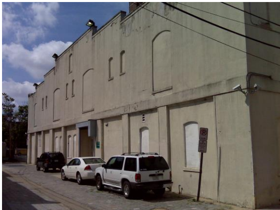
Old stables at 1300 Naylor Court serve as the District's Archives.
