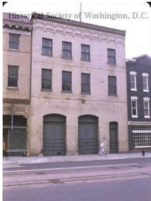
Figure 8 By Congressional legislation, the AOI was "offered" the old No. 5 Engine House on M Street just west of Wisconsin Avenue if the AOI met certain conditions.
