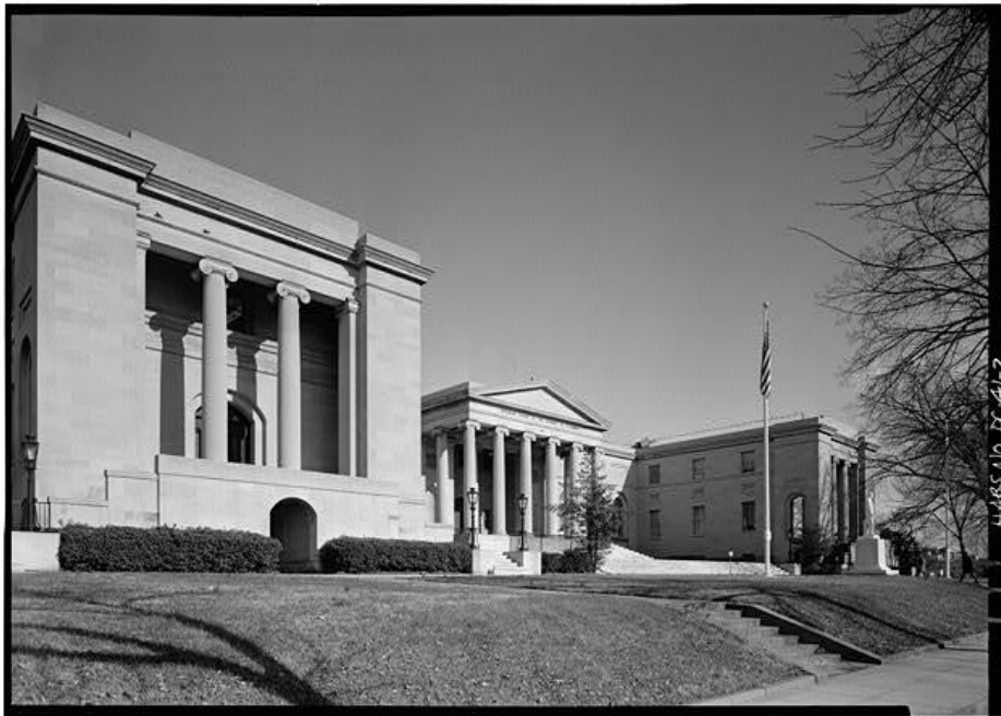
Figure 1 Old DC City Hall now the Court of Appeals (from HABS).
