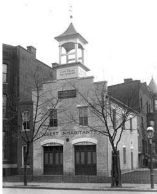
Figure 5 The old Union Fire House served as AOI's headquarters from 1909 until the property was sold to the World Bank and International Money Fund in 1955.
