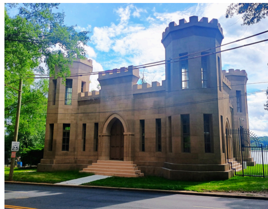
As originally noted in our Spring 2024 Newsletter, AOI was in the forefront of efforts to hold the Army Corp of Engineers' feet to the fire in their restoration of the Washington Aqueduct's Castle Gatehouse. The finished result, looking as good as new, debuted this spring – job well done!
