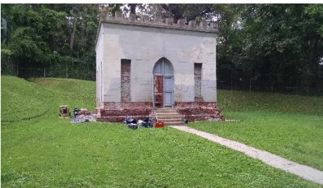
Figure 3 City Tunnel West Shaft Gate House under rehab
