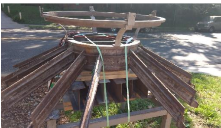
Figure 8 New skylight/oculus for Inlet Gate House
