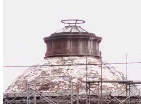
Figure 4 Inlet Gate House under renovation
