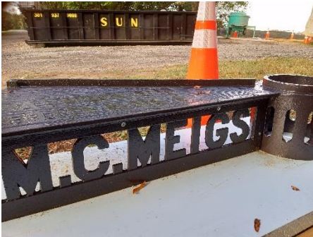
Figure 7 New stairs for the Meigs vault
