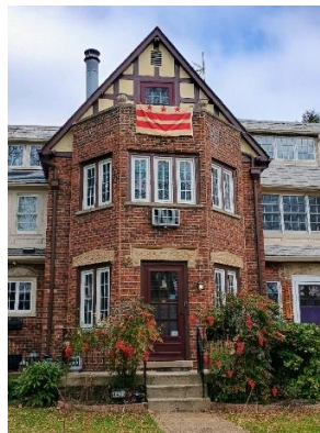
Figure 26 Showing my DC pride at 4425 Greenwich Pkwy., NW
